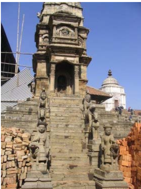
A Buddhist temple that's under construction in Nepal.
